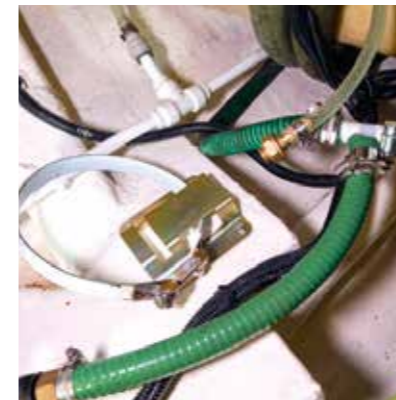
The T-piece, white tubing and bracket for the accumulator all in place
