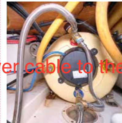
Thermostatic mixer valve (top) in place on the cylinder's hot water outlet. Note the blue power immersion heater power cable that goes into the black cover: this must be isolated before starting work
