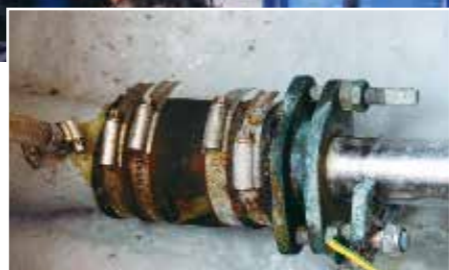
LEFT Imagine loud vibration and smell of burning. A carbon brush that was fitted to connect to the prop shaft for galvanic protection, damaged a brass bolt when a Nylock nut loosened
