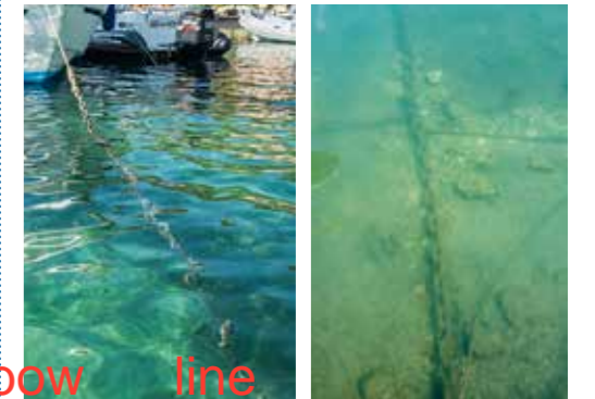
The bowline from each boat is connected to a chain. This in turn is connected to a bigger chain that runs parallel to the dock. The big chain is secured at either end to the dock or a large lump of concrete
